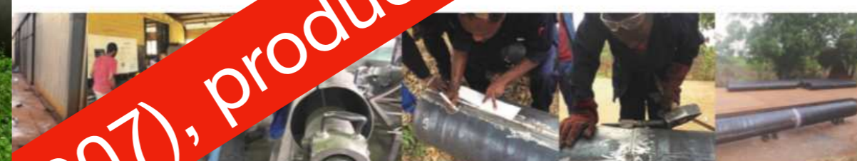
the tube sections Rolling and welding tube sections Visual inspection of longitudinal welds Joining two tubes together Quarter-lengths done!
