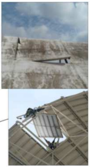
Surface panels repaired and refurbished
