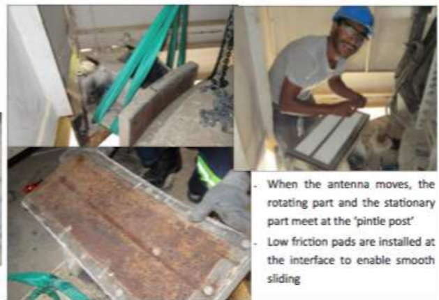
Replacement of pintle pads
