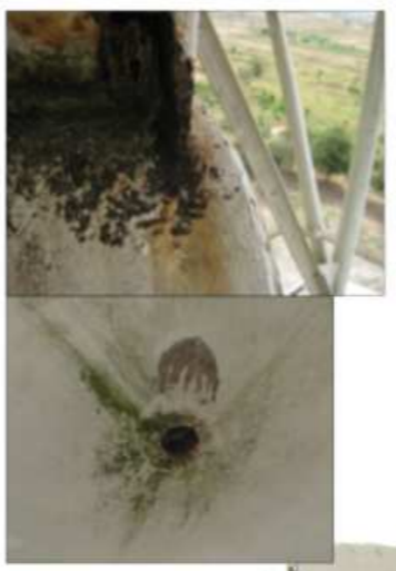
Rust, algae removal and painting
