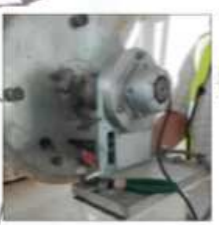
Azimuth and Elevation encoders replaced
