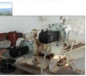
New motors and control system
