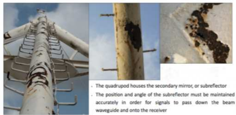
Subreflector support ("quadrupod") legs replaced
